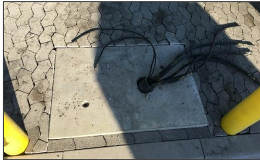
Figure 15: UU foundation preparation
